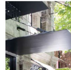
SP Steel Plate Paint Finish Location: Rooftop bar awning
