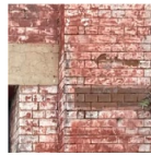
BR-E Brickwork - existing Existing paint stripped Location: Existing facades
